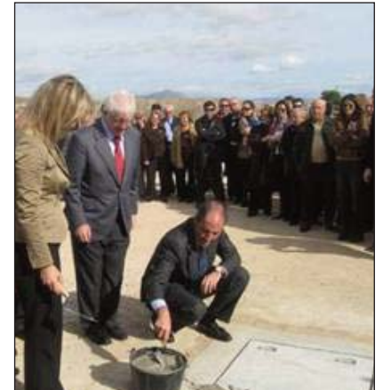
Francisco Camps lays the first stone of the new wastewater treatment plant.
