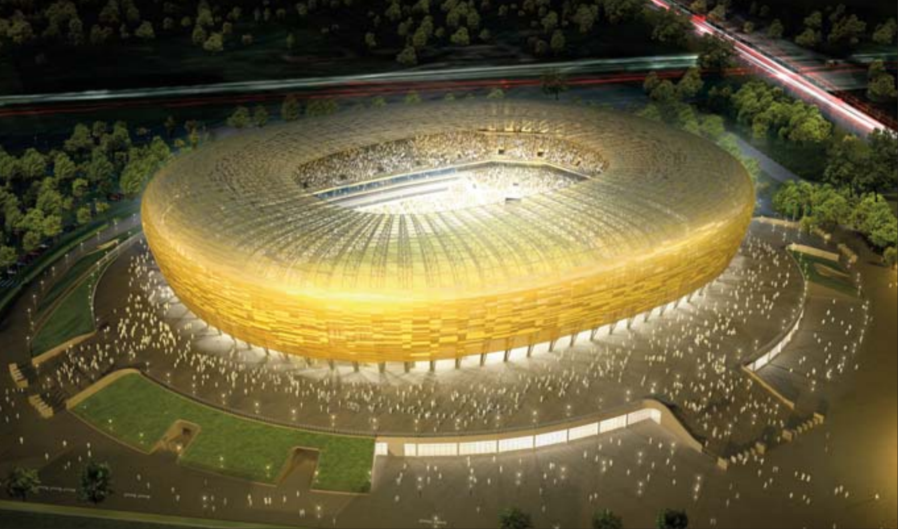
New Baltic Arena project in Gdansk.
